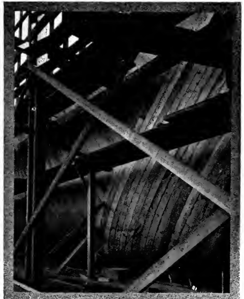
The diagonal planking used on the hull of the steamer being built at the Kiernan & Kern shipyard.
